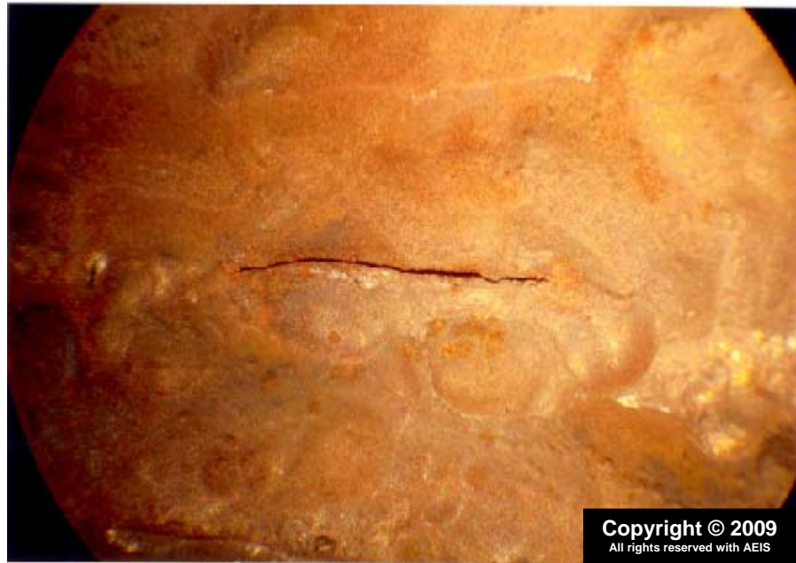
Figure 3: Crack Lips on the Inside Surface
